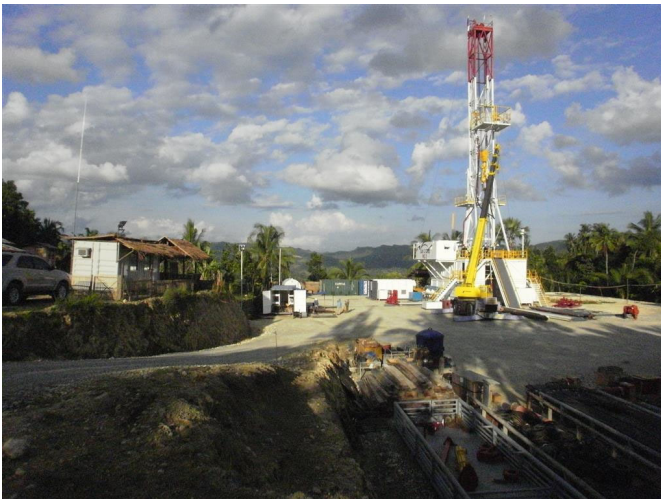
Company owned drilling rig located in Cebu
